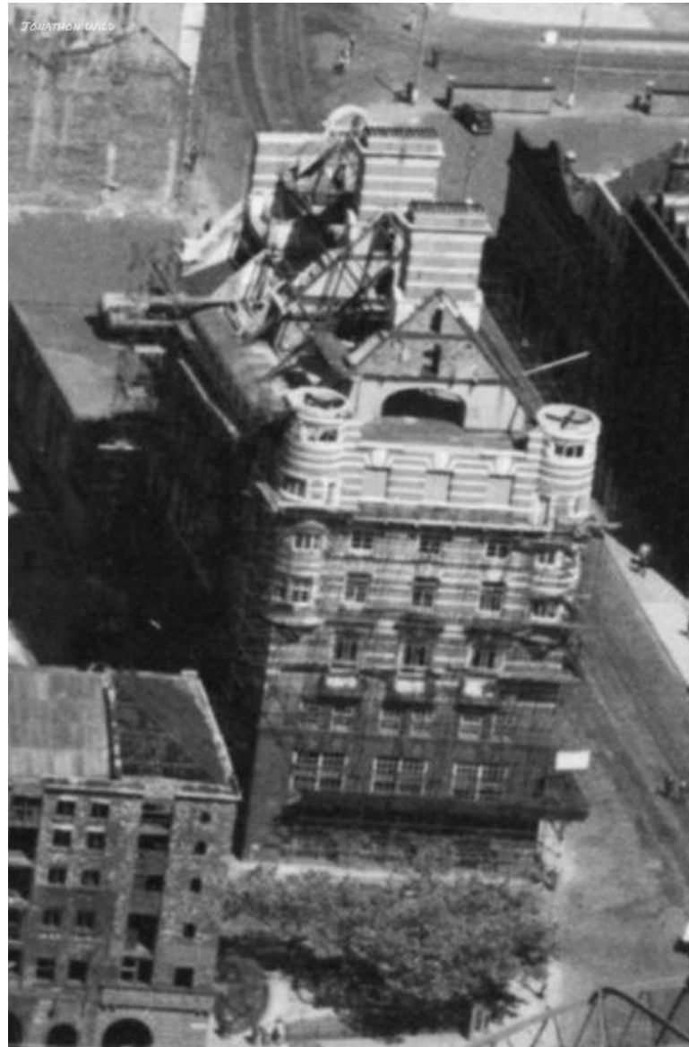
A view of the 1946 refurbishment show the removed gable end including some of the front wall to rebuild on solid foundations.
