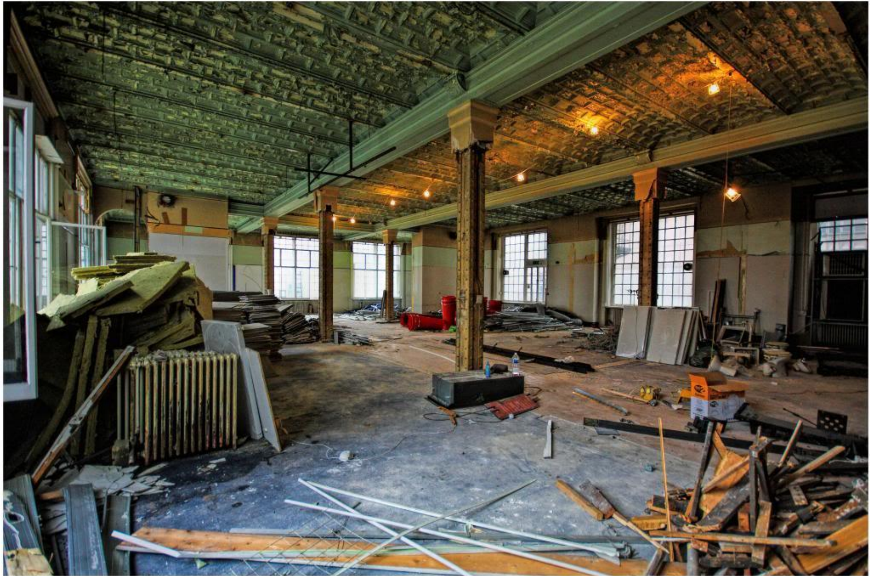
In the above view of 2014, we see the Grand Hall now being uncovered after years of neglect. The iron beams rediscovered once again as well as the fire-resistant ceiling!
